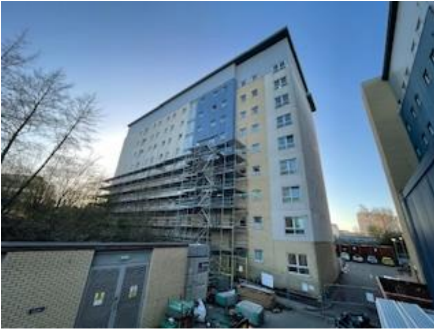
Phase 4 scaffolding ongoing
